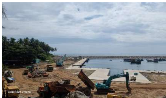
Construction of travel lift bay
