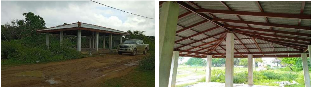
Renovaition work of aucton hall & Net mending hall Nachikuda Kiranchi
