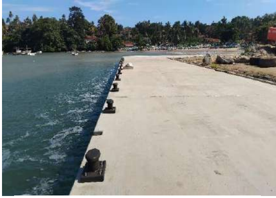
Construction of the quay wall
