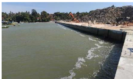
Construction of the quay wall
