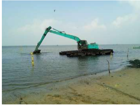
Cleaning of the Existing Access Poonakary
