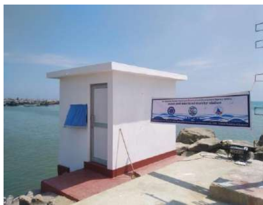
Figure 13. Newly Constructed Sea level Monitoring Station at Dondra Fishery Harbor
